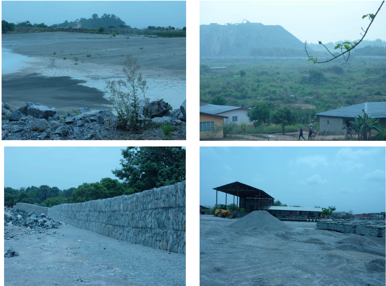
Figure Two. Koidu Kimberlite Project. Top left. Disused slimes dam. Top right: Waste rock dump steeply adjoining lease boundary – note the lease boundary rock wall at the foot of the dump. Bottom: Reuse of waste rock in wall construction (left) and brick construction (right).
