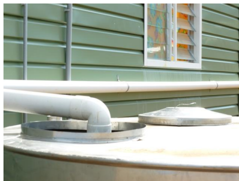
Figure 5: Incorrect Installation of Rain Water Tanks
